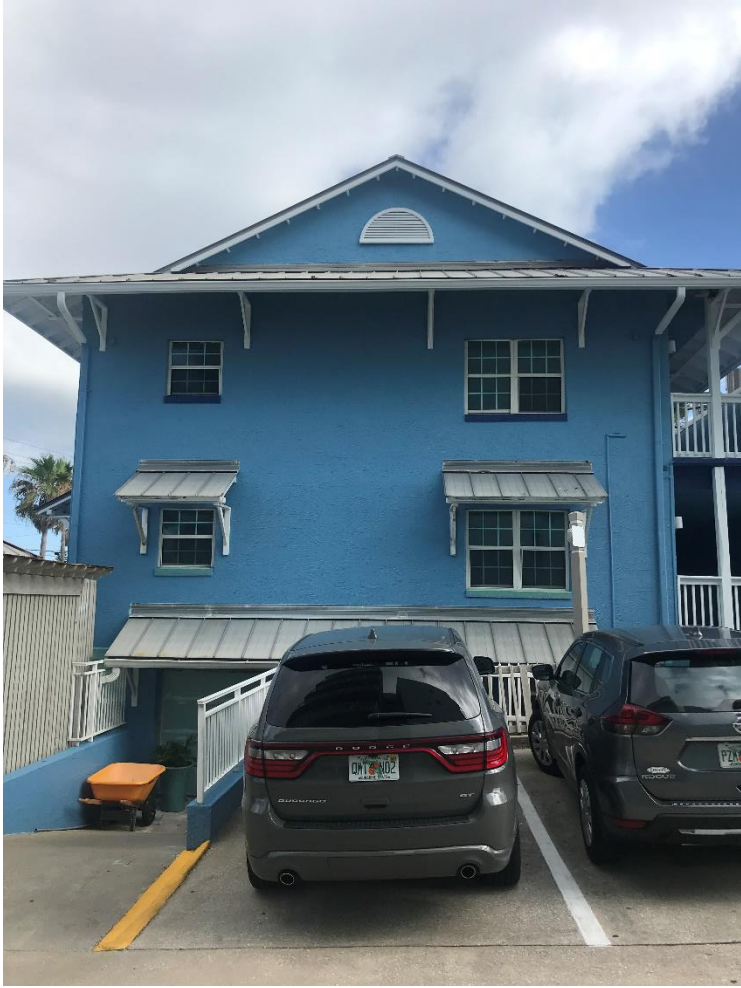
Traveler Building – above maintenance shop
