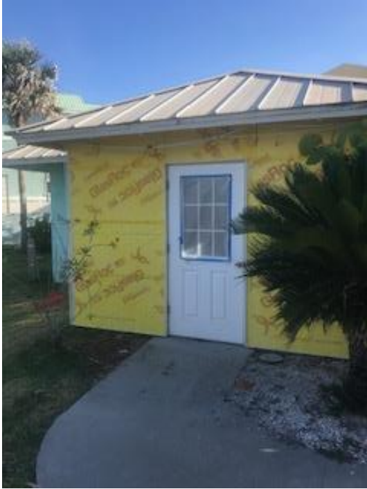
Mesh rough in – Thatch laundry room
