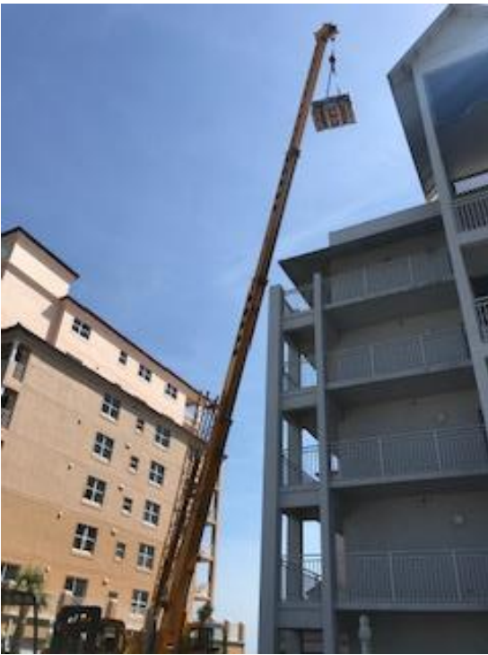
Royal Palms building – roof materials being put on roof.
