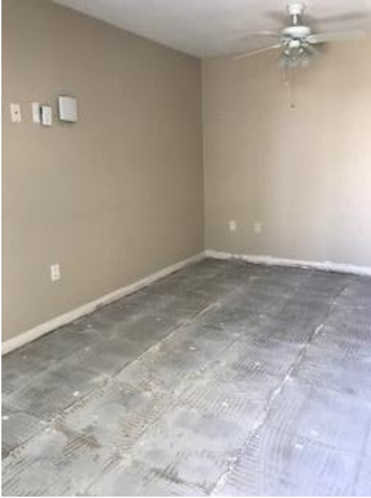
Floor tile removal in the bungalow
