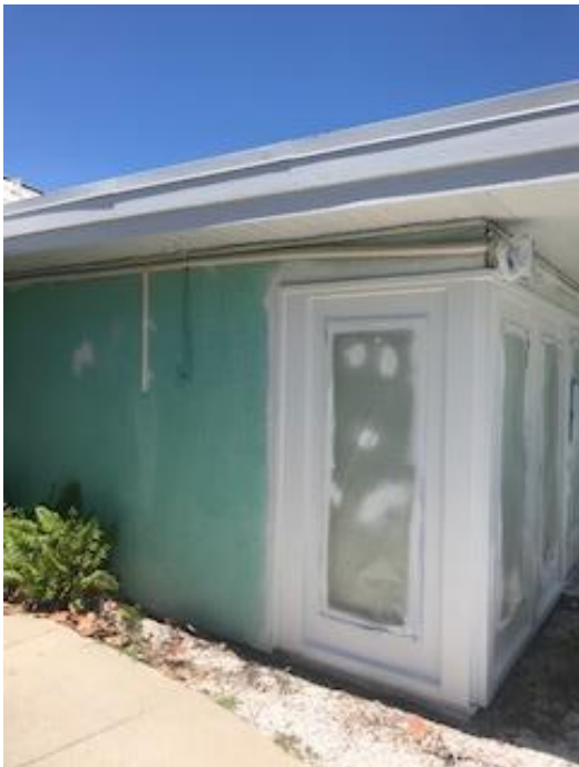
Taping off and soffit painting
