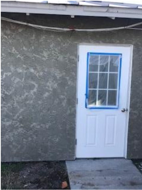
Thatch laundry room – stucco repair
