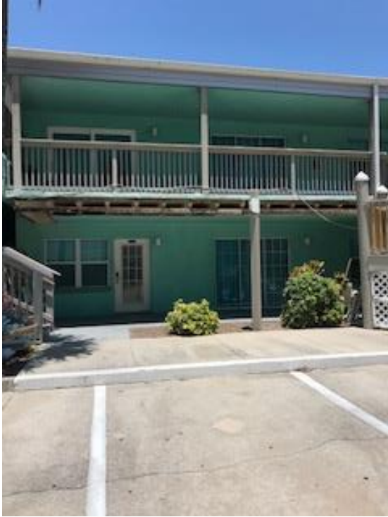
Traveler – preparation for stucco repair
