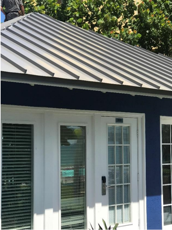
New metal roof on Thatch
