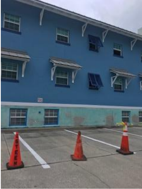
Traveler Building – west side
