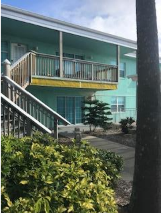
Traveler Building – front side stucco repair for inspection
