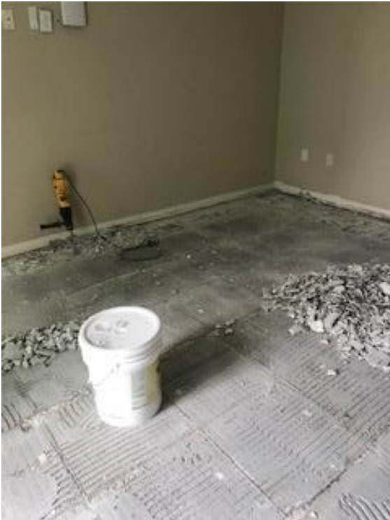
Floor – Thinset removal
