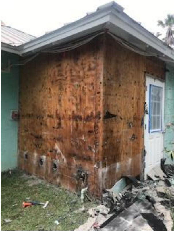
Demolition for stucco repair
